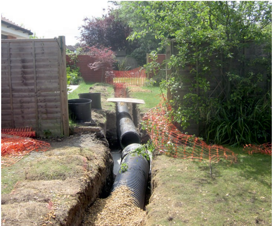
Drainage works in progress in Sole Farm Avenue
