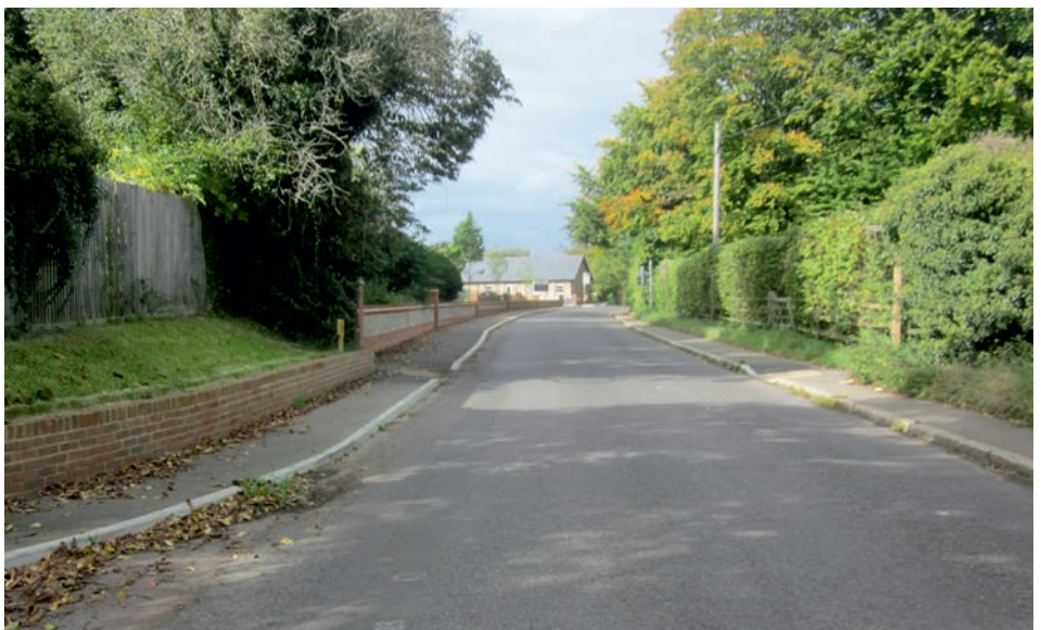
New footway on Rectory Lane at the Gracewell Care Home
