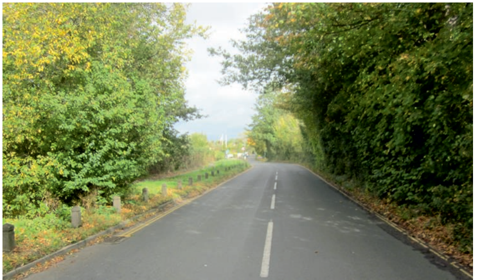
Vegetation has now been removed on Lower Road improving sight lines.
