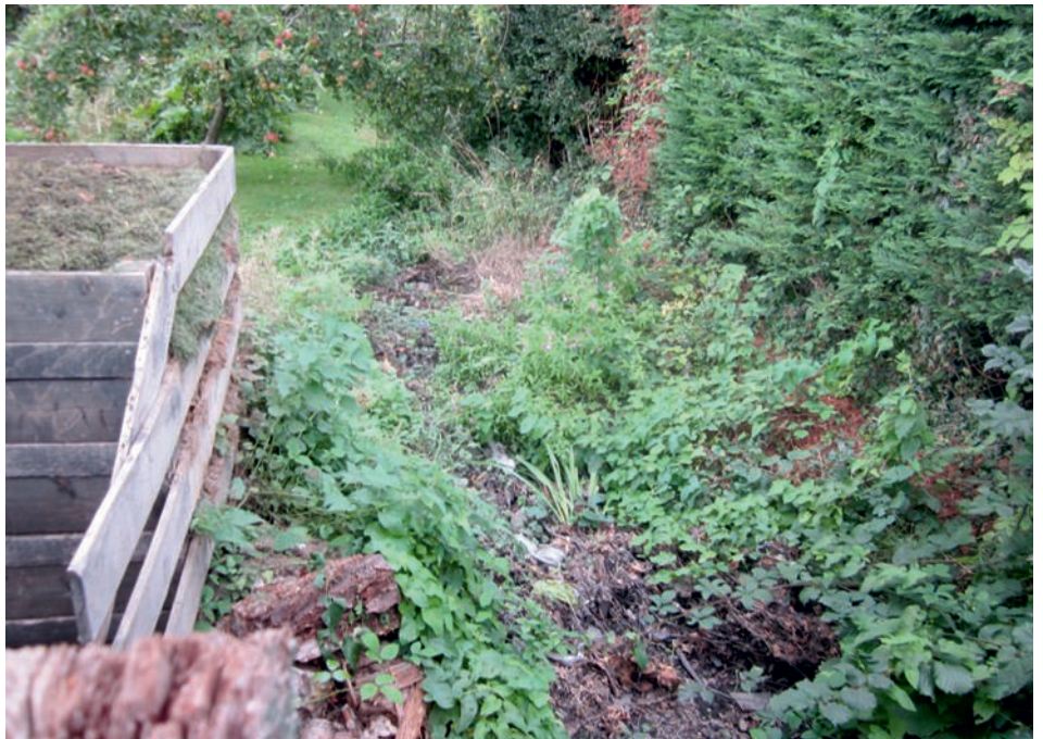
Overgrown length of ditch at Childs Hall Road.
