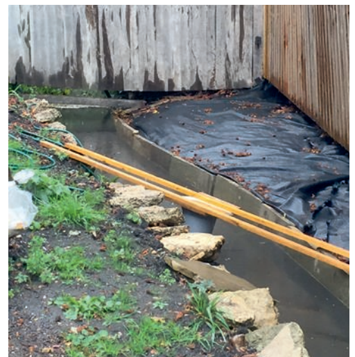
Ditch passing through a resident's property on Lower Road about to overflow following heavy rainfall.
