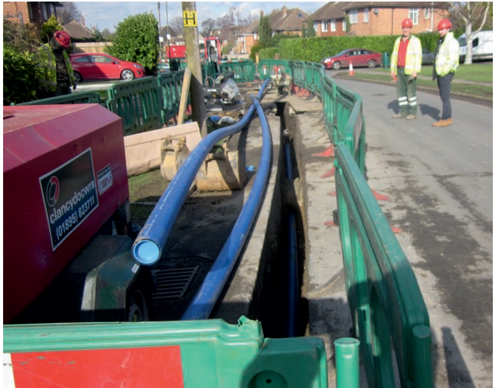
Replacement water mains by Sutton & East Surrey Water Company.
