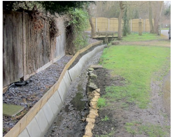
Well maintained ditch north of Lower Road
