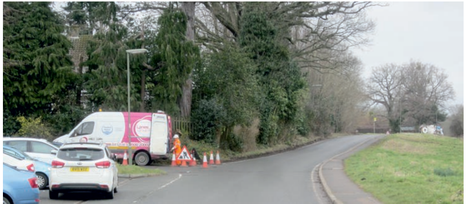
Thames Water contractor clearing the drains in Little Bookham Street.
