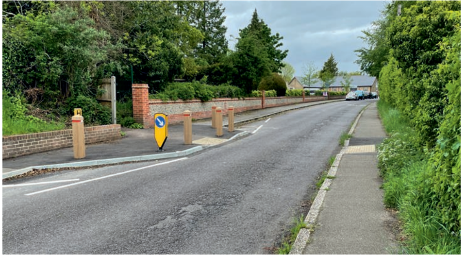
Recently completed Build out in Rectory Lane to provide a safe crossing point for pedestrians.
