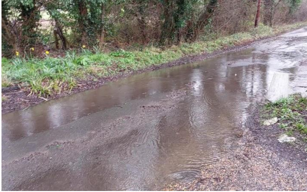
Figure 2 - Water flowing down Water Lane 2 nd March 2024
